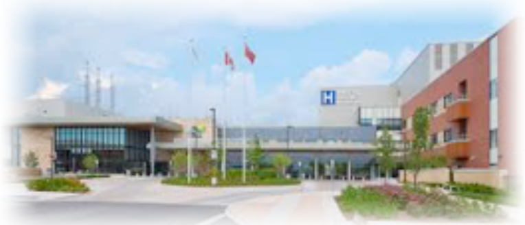
Milton District Hospital
