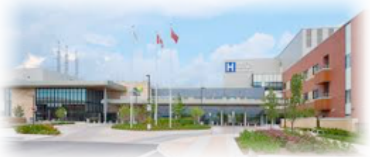
Milton District Hospital
